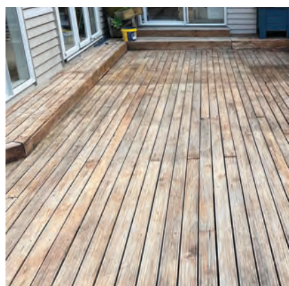
Deck after wash and scrub
