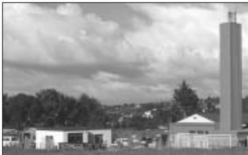
The tall chimney of the Long Bay College boiler house, which has been a landmark for 30 years, is due to be demolished.
